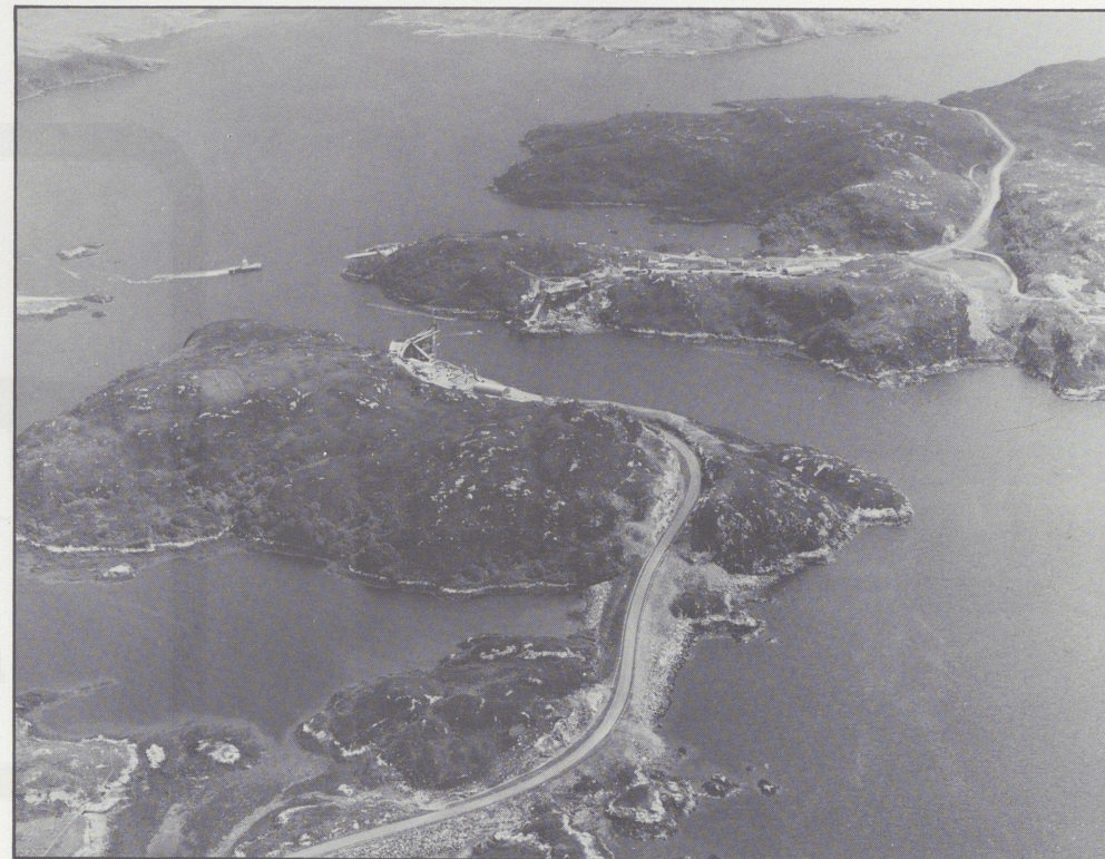
An aerial view of the site.
