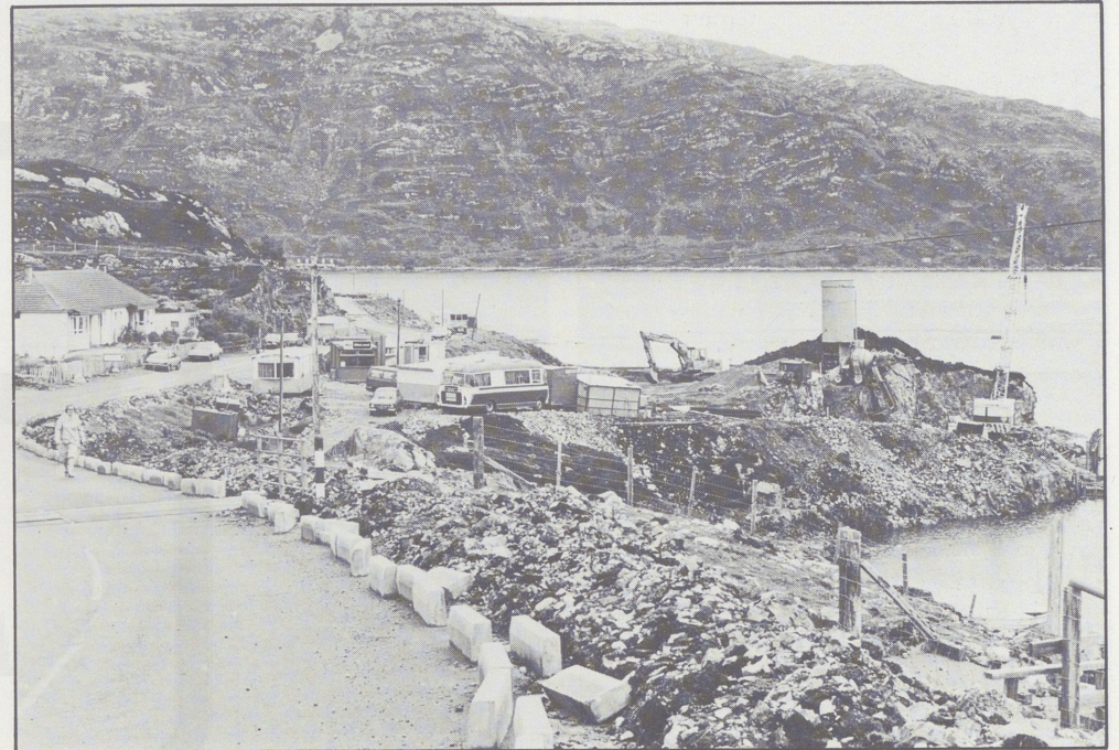
Village footpath and Fishery Jetty under construction.
