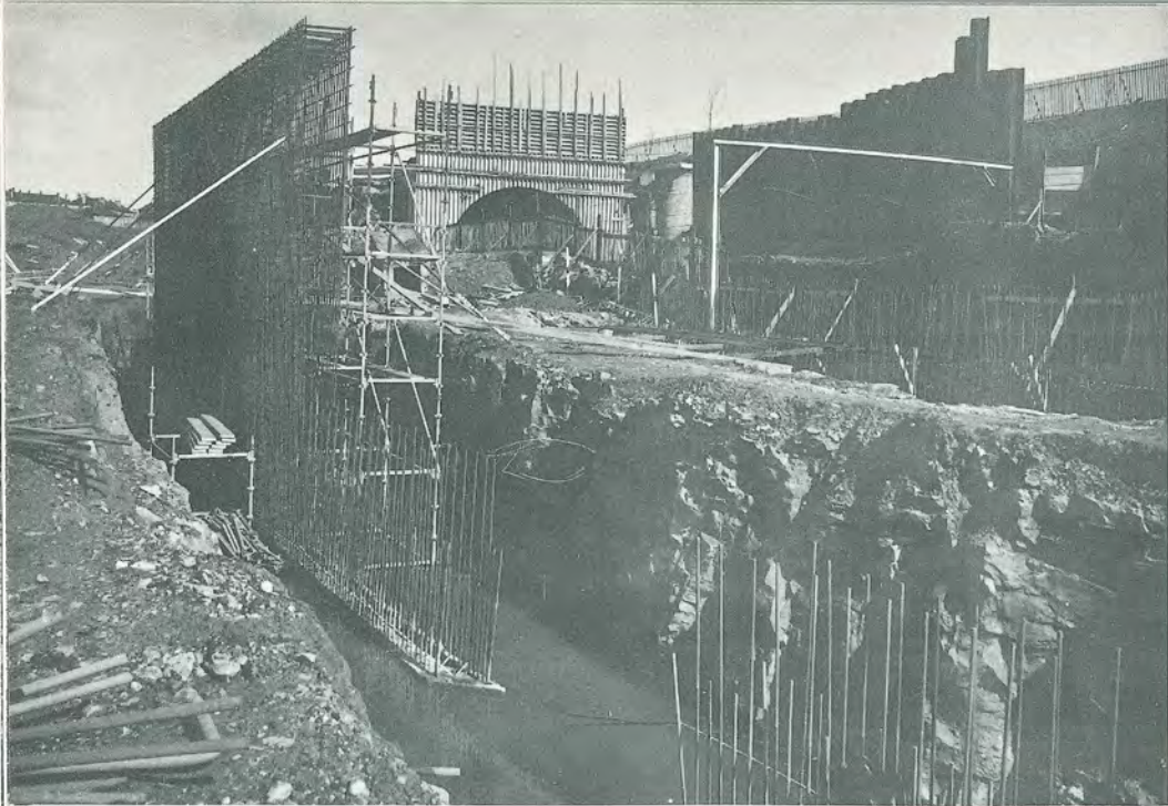
Blochairn: New portal at south end of railway tunnel.
