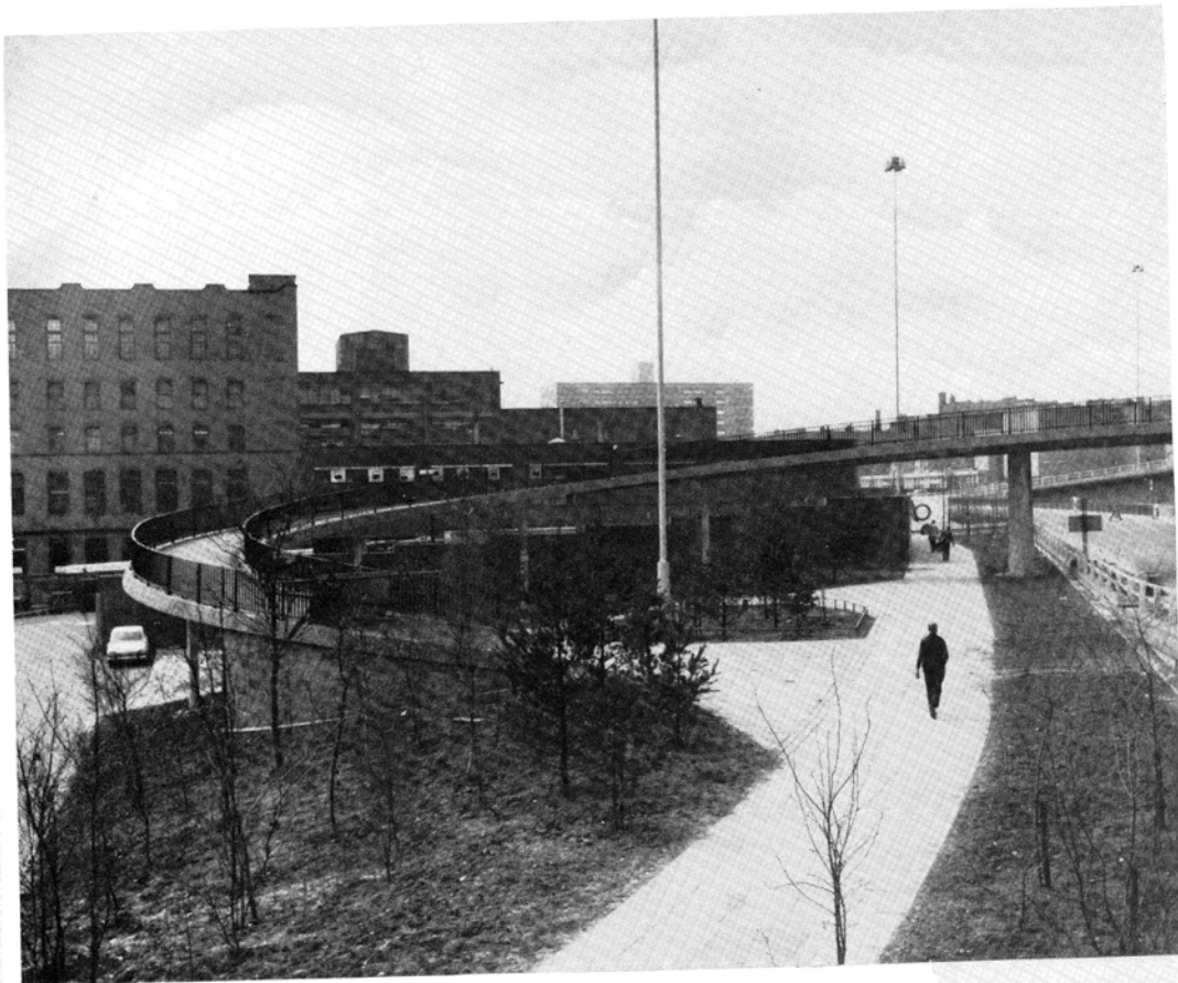
Arrangement for pedestrians at Stobcross Street
