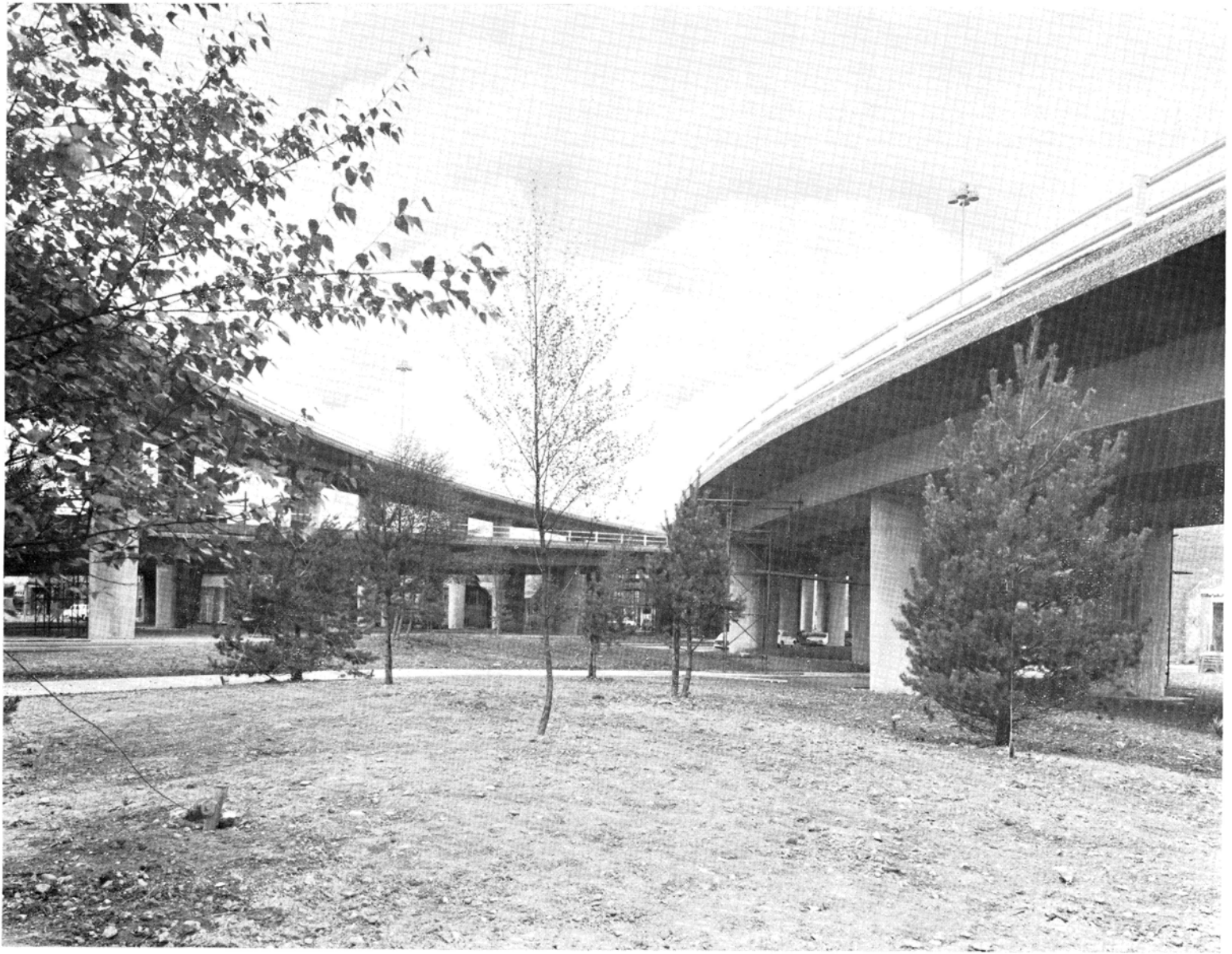
3-level interchange at Carnoustie Street showing soft landscaping
