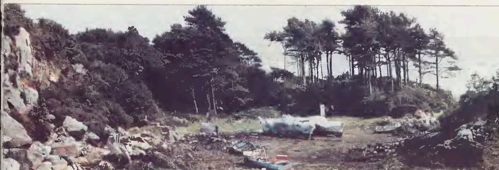
◀ Looking east along the proposed road line below Lochalsh road before and after construction
