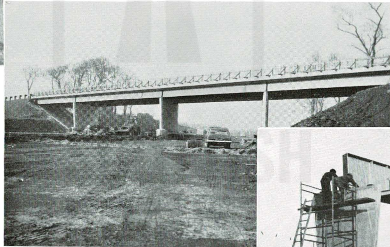
Sandyford Bridge—Reinforced Concrete “ Box ” Design
