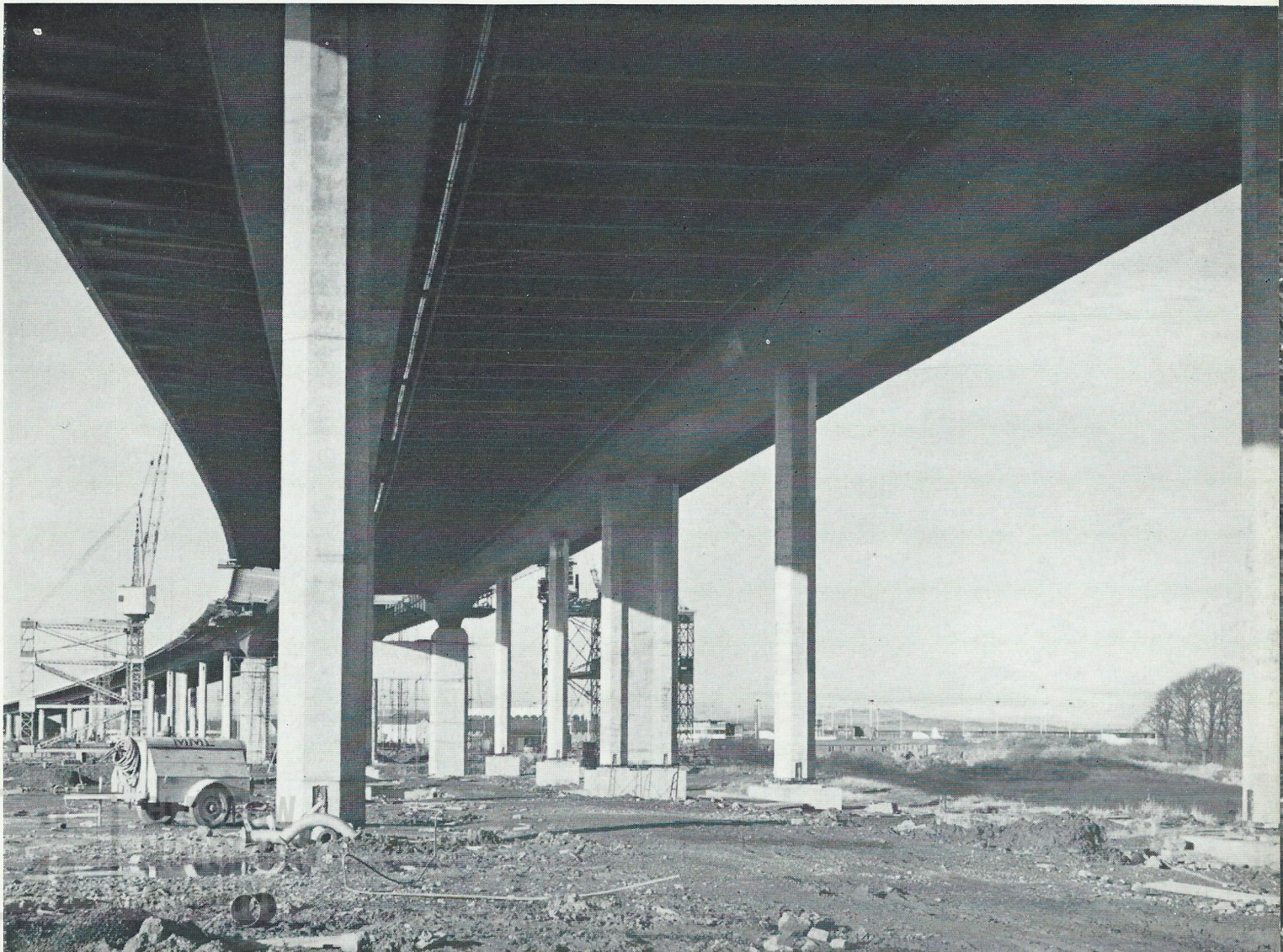
The slender octagonal rocker columns supporting the six lane motorway.
