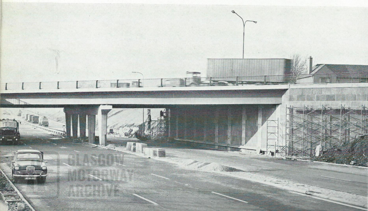
Bridge carrying Paisley-Renfrew road.
