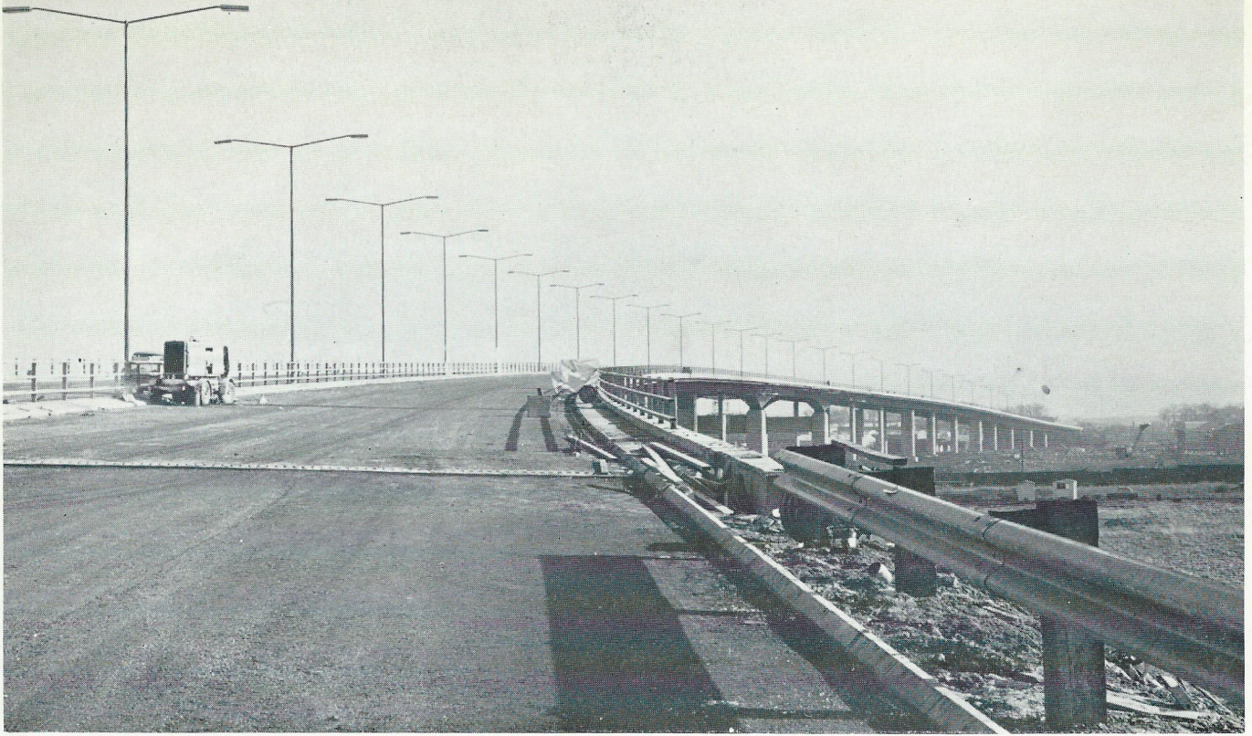
Viewed from the Airport end the curved viaduct nears completion.
