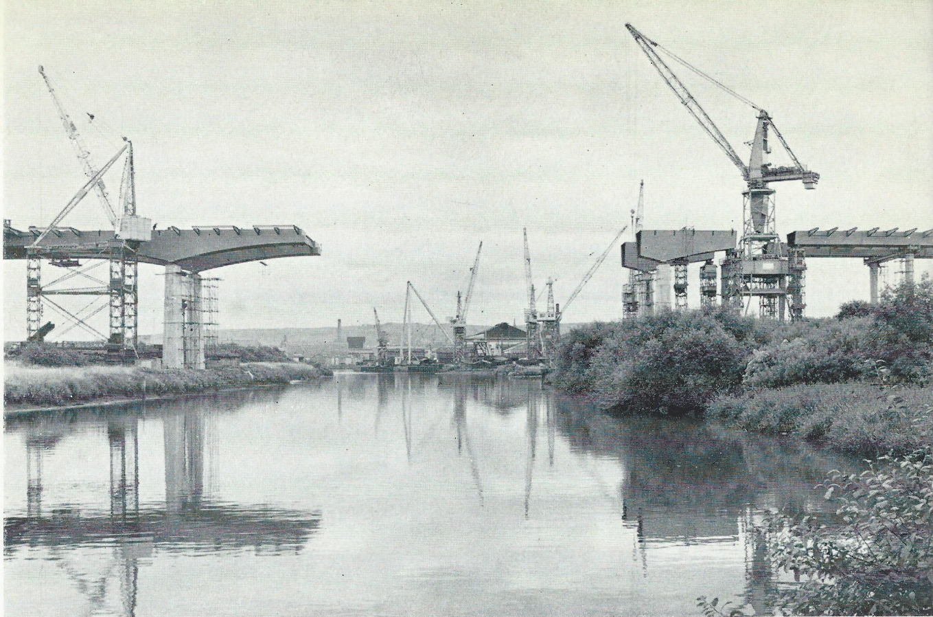
Erection of main span steelwork in progress looking upriver to Paisley.
