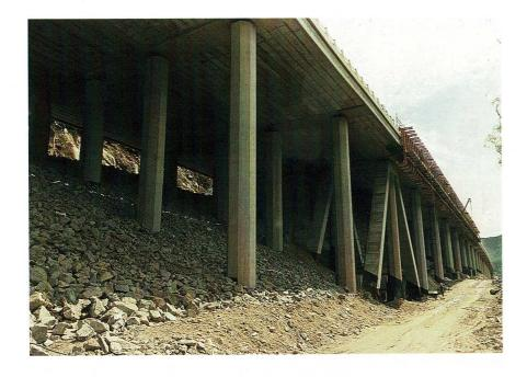
The structural option was developed in detail, each viaduct consisting of short 15 metre deck spans constructed with precast tensioned beams joined with in situ concrete over dual octagonal columns, each seated on 4 metre square bases founded on rock.
