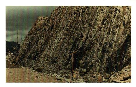
The rock exposed on the uphill side of the viaduct was excavated by pre-split techniques (parallel holes drilled and pre-blasted at the face of the cut) to minimise blast disturbance to the standing rock face.
