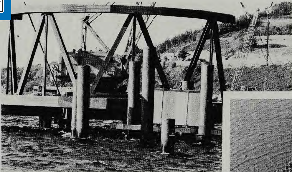
Waling being reassembled on location
