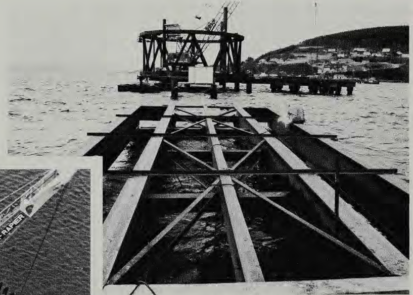
South Approach access jetty under construction
