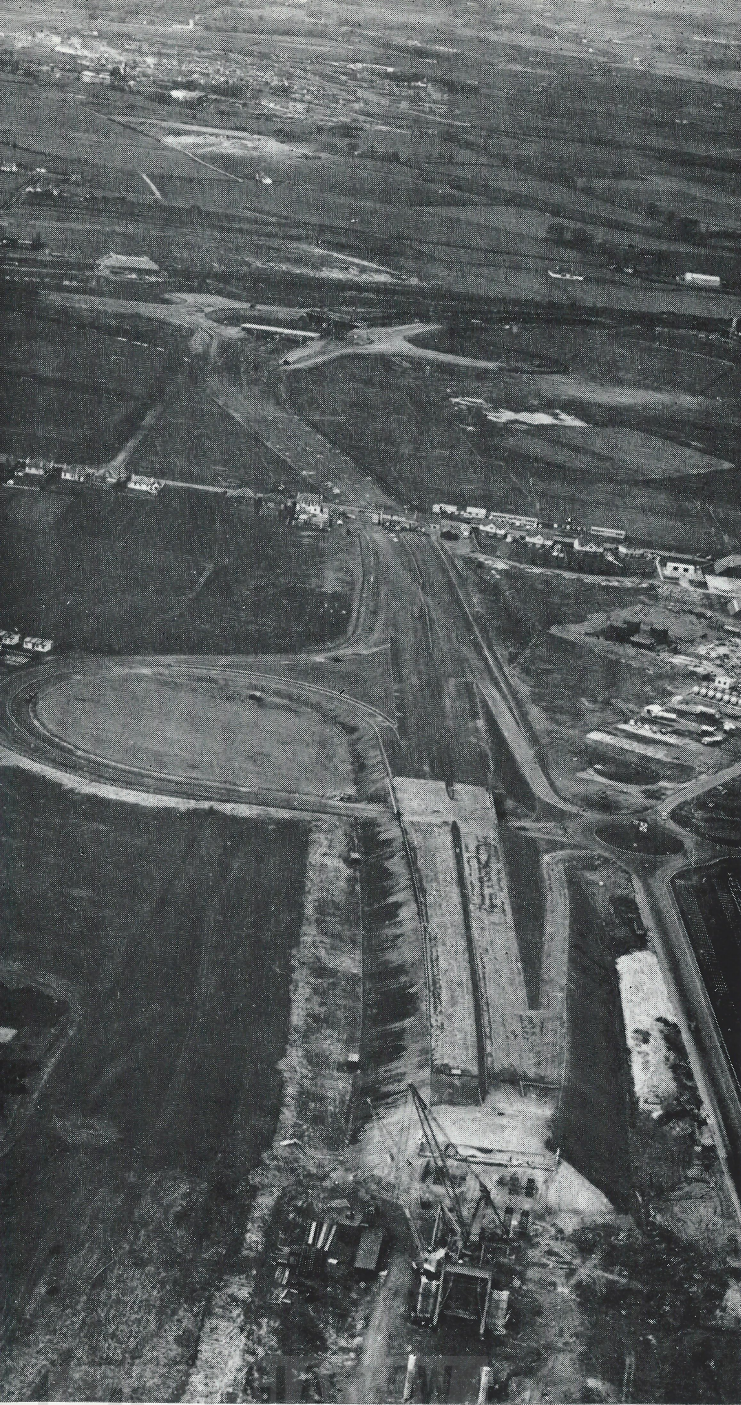
Interchange giving Access to Glasgow Airport with the St. James Interchange at top of photograph.
