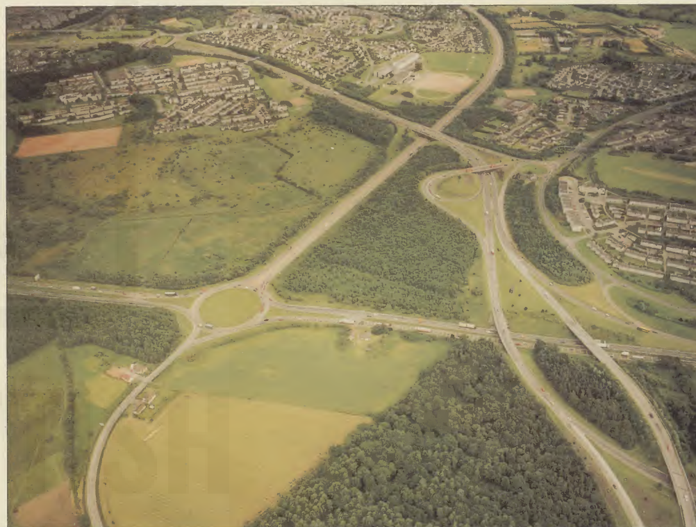
Auchenkilns Roundabout and Low Wood Interchange
