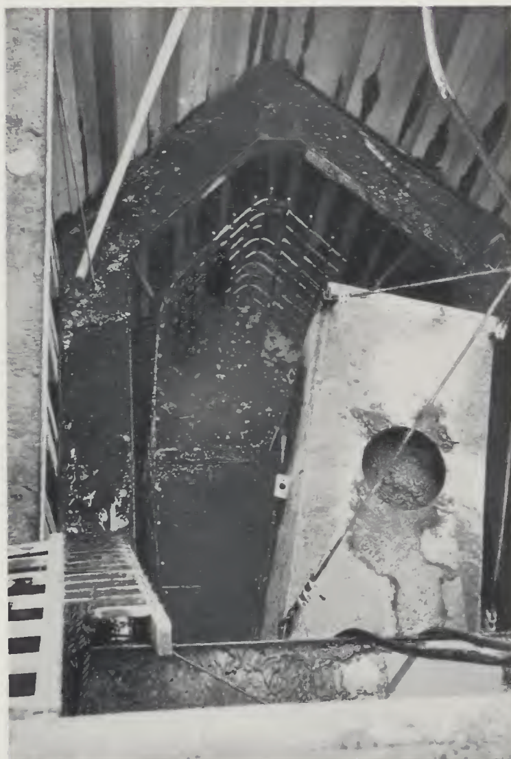
Below water the cofferdam itself formed the mould for each pier. Near the surface shuttering was set to produce the smooth boat-like outline in the centre photograph. Shuttering was then set for the twin columns, one of which is shown on the right.
