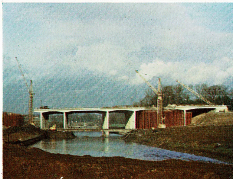
Top left Sub-structure and column supports for new Avon Bridge.
