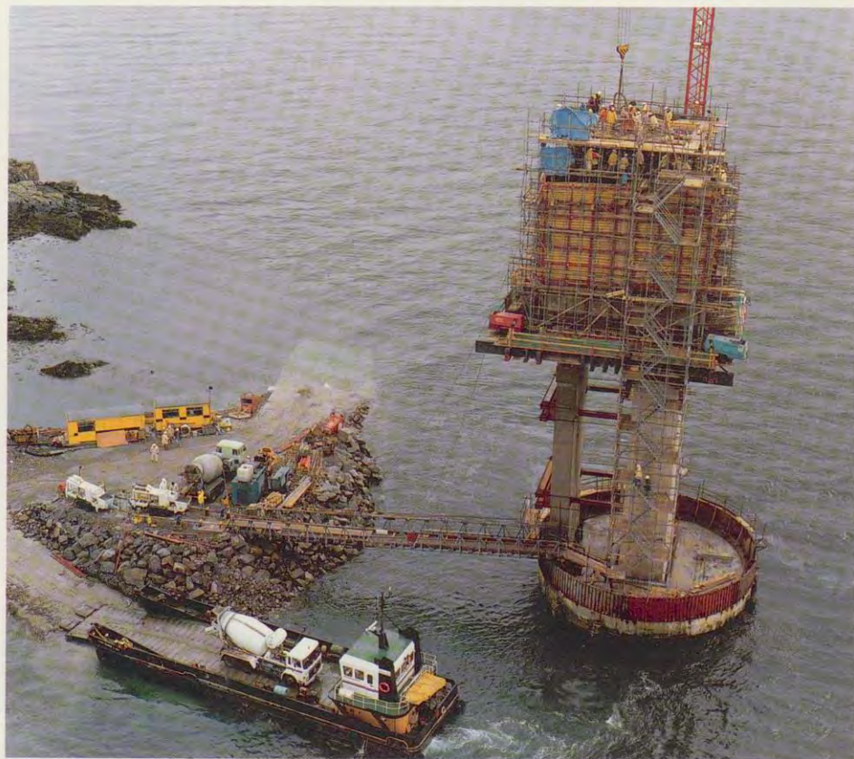
Building the pier table above the foundation
