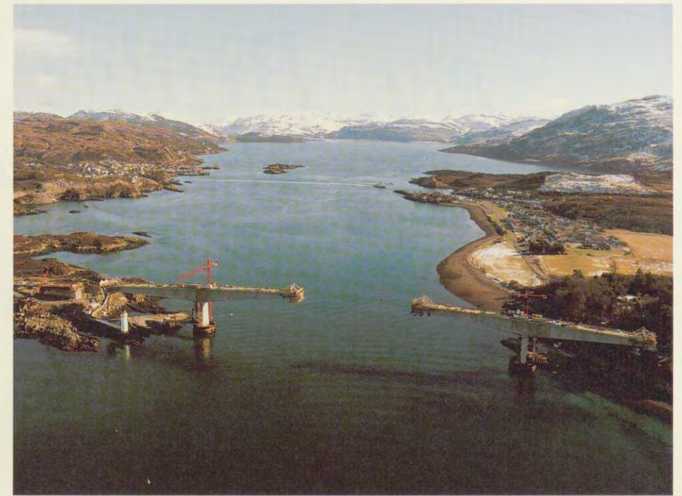
The Skye Crossing under construction
