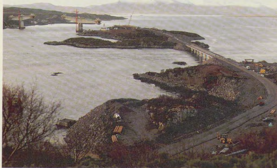
Construction of the approach to the Carrich Viaduct
