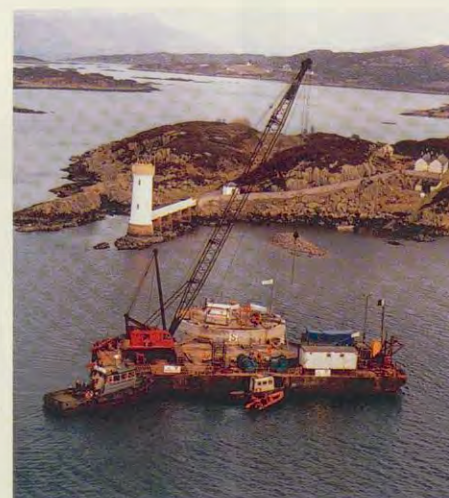
Placing the south caisson
