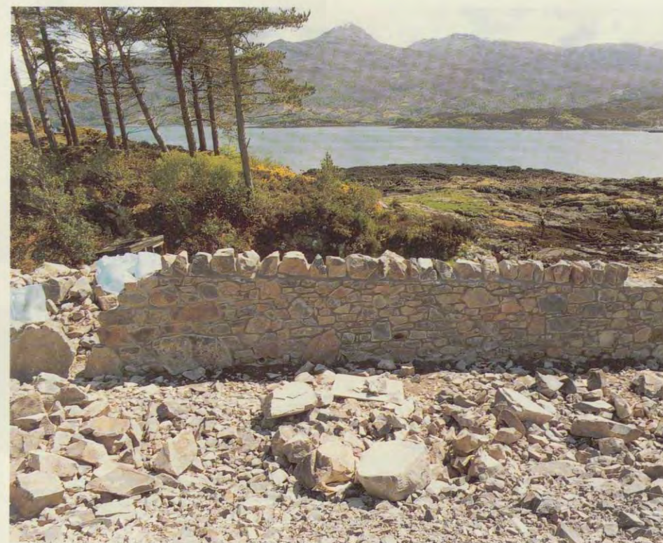
Construction of the Otter Wall
