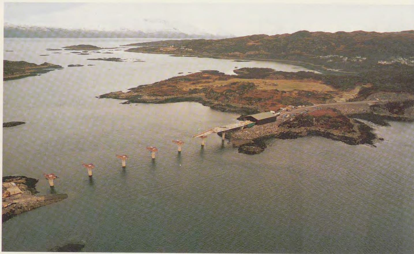
Building the deck of the Secondary Bridge
