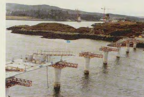
Building the Carrich Viaduct
