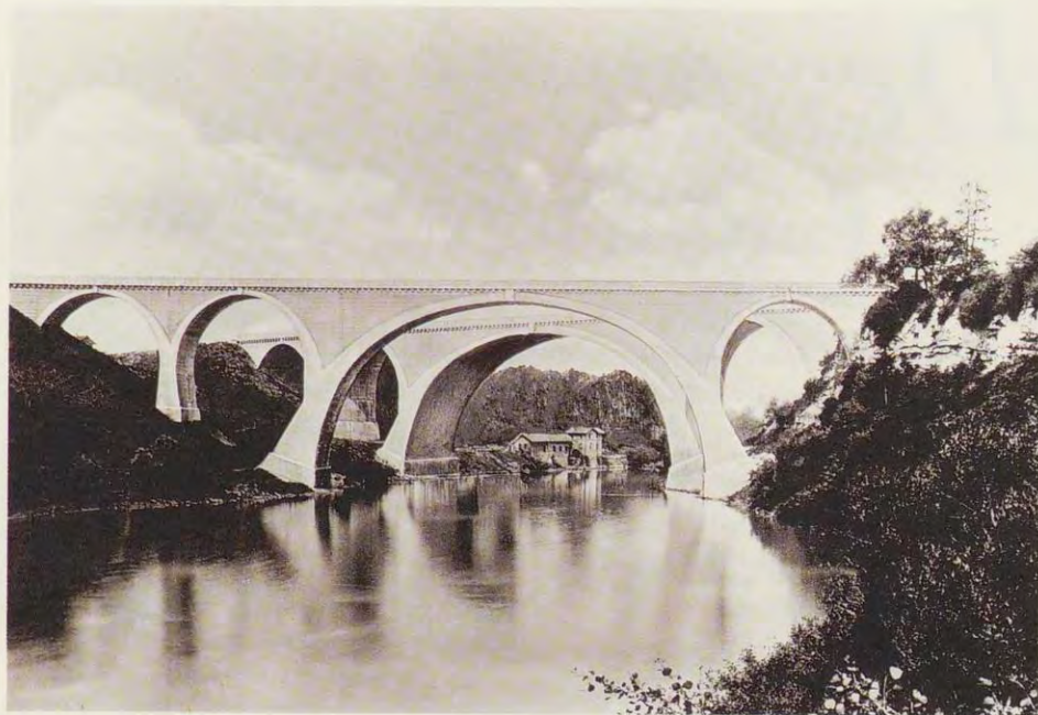
An early Dywidag bridge over the Iller, Kempten 1904 / 1906
