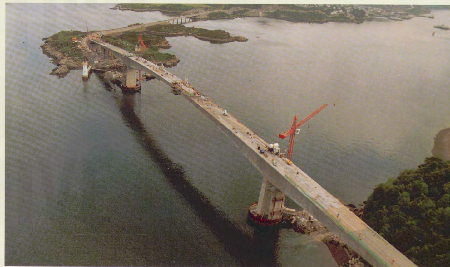
Completing the main span
