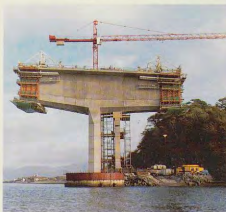
The balanced cantilever process
