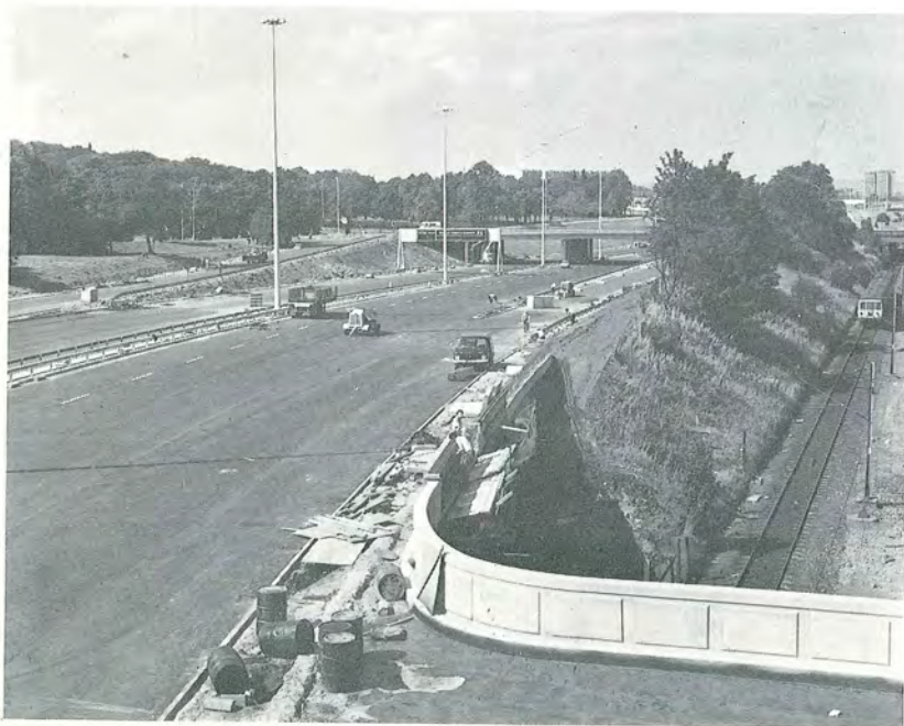
Stage 1 viewed from Beech Avenue Footbridge looking West.
