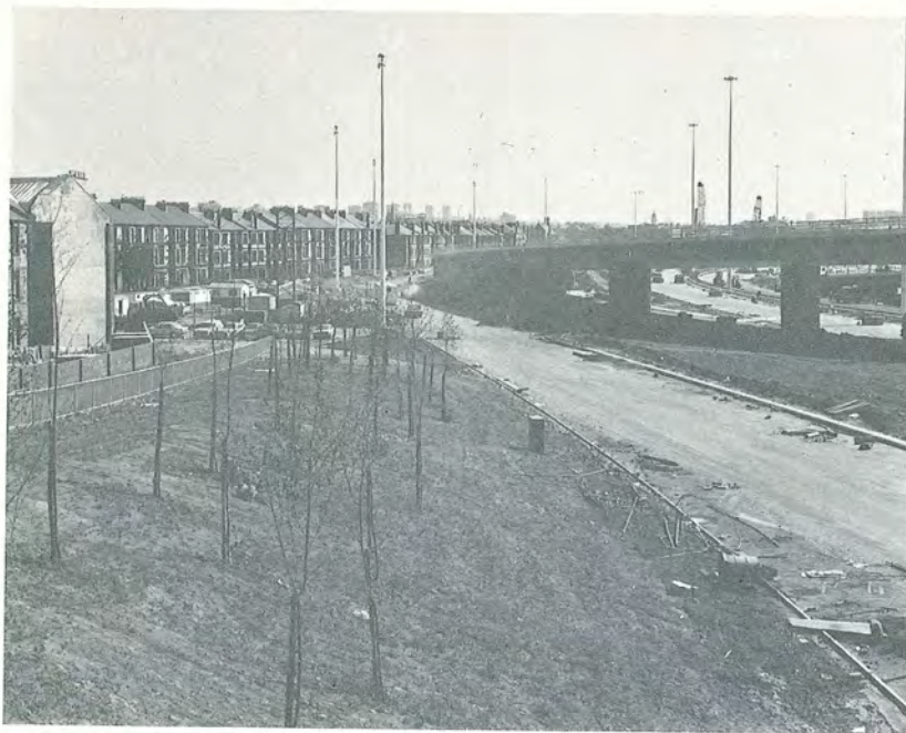
Stage 1 viewed from Kirkwood Street Footbridge looking East.
