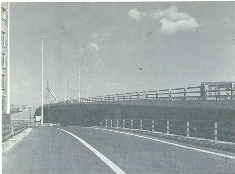
Scotland Street Viaduct viewed from the off ramp to Seaward Street.
