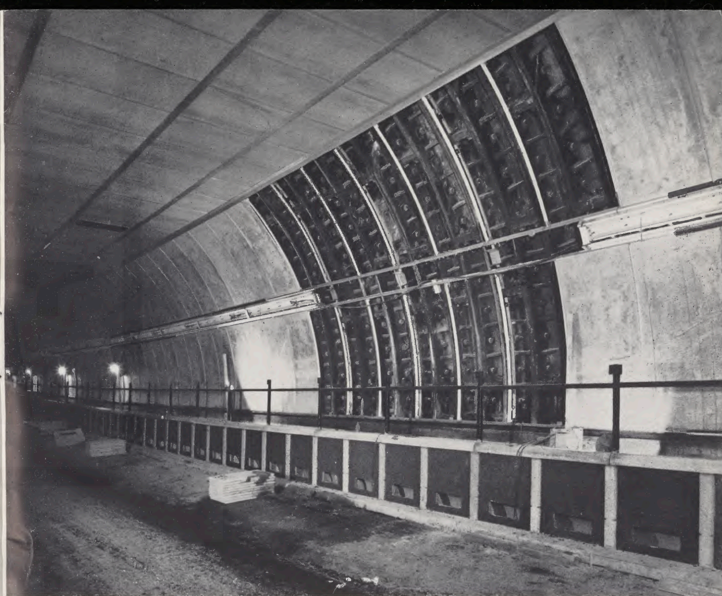
The last view of Tunnel Segment Castings in the Clyde tunnel before they are clad.
