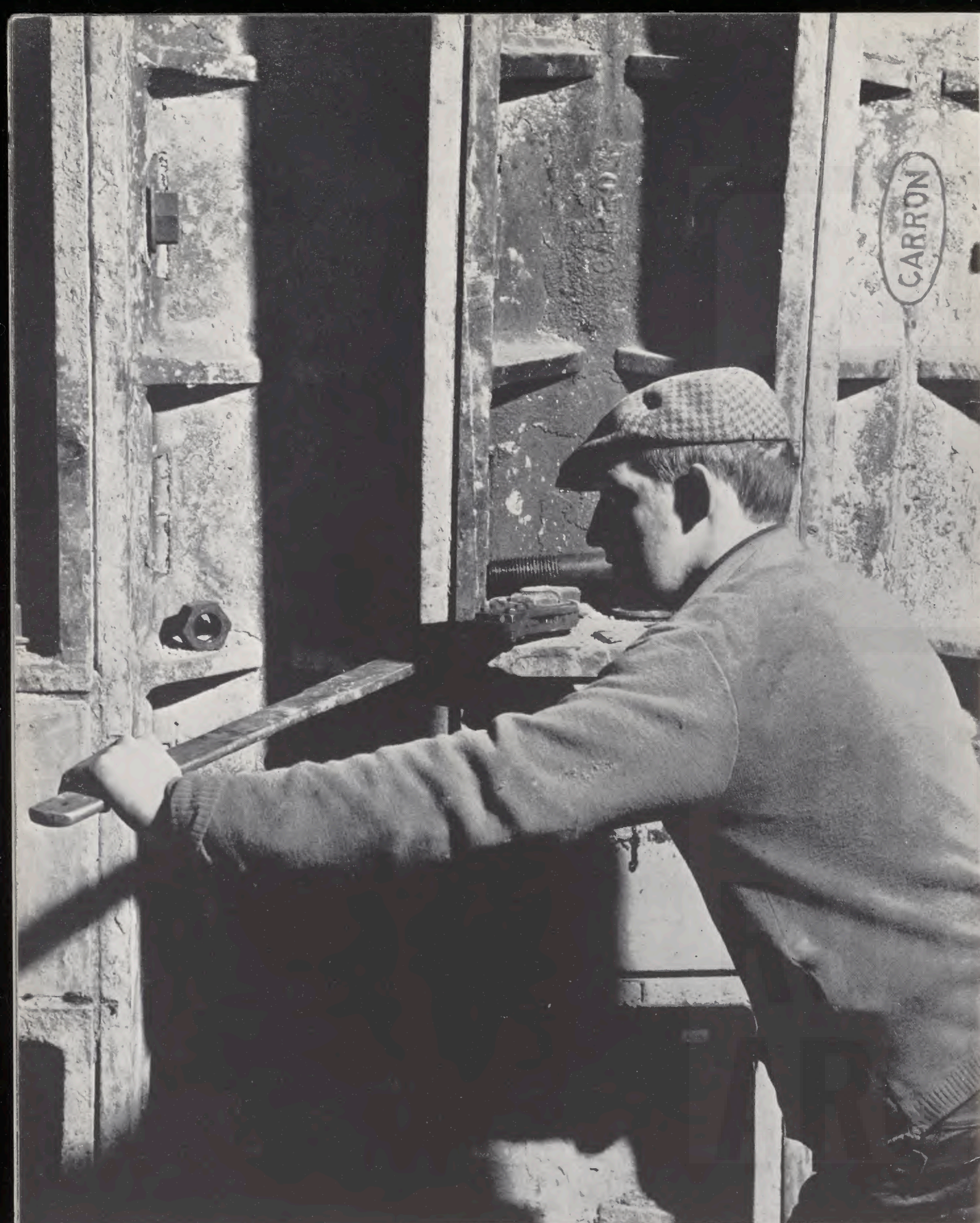
Tightening radial joints of segments.
