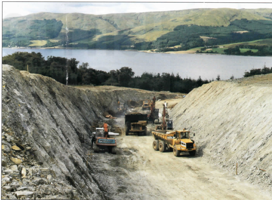
Construction of a rock cutting on Northern Access Road.
