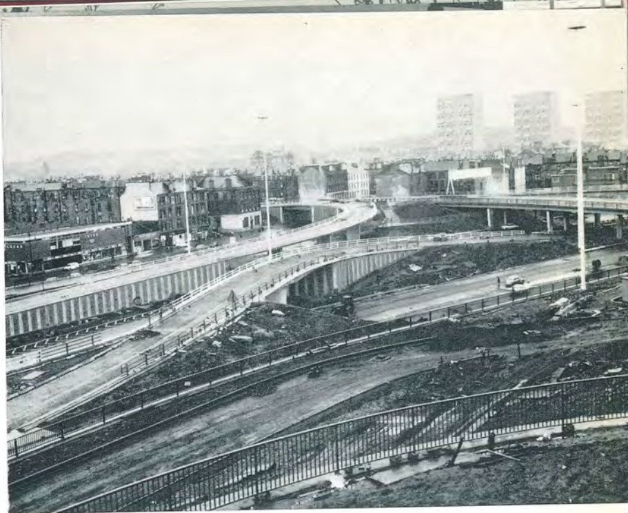
St. George's Cross Interchange
