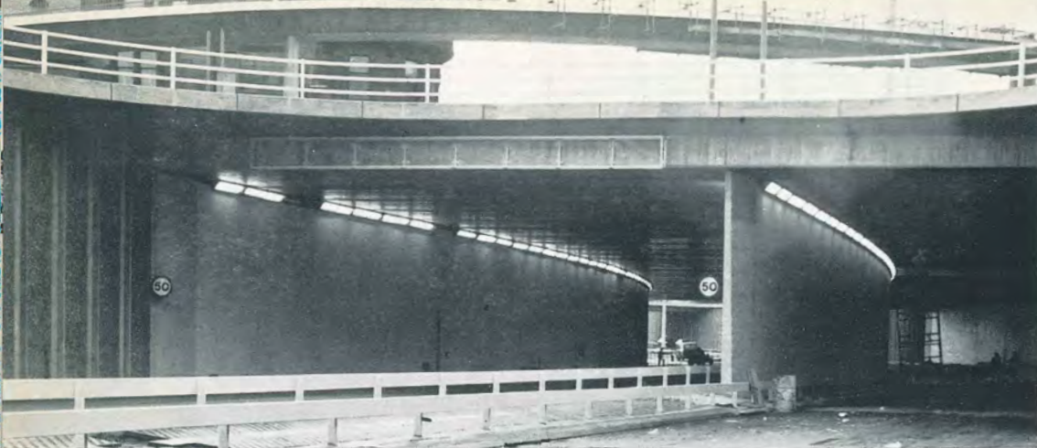
Charing Cross Tunnel—North Portal
