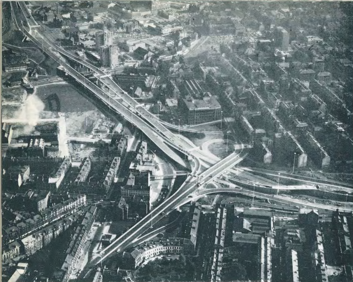
Plate No. 1 Aerial View of Woodside Section
