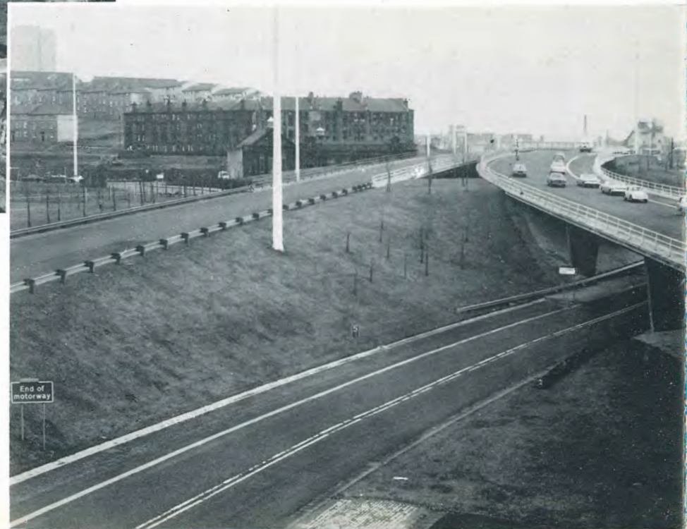
Plate No. 4—Looking East from Baird Street Bridge
