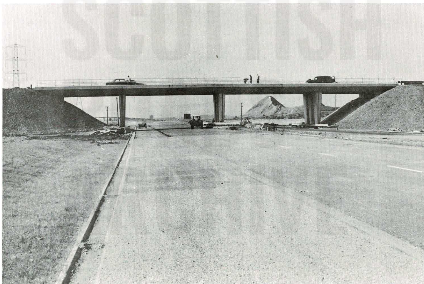
ILLUSTRATION NO. 3 WESTERTON ROAD OVERBRIDGE (BRIDGE NO. 2).
